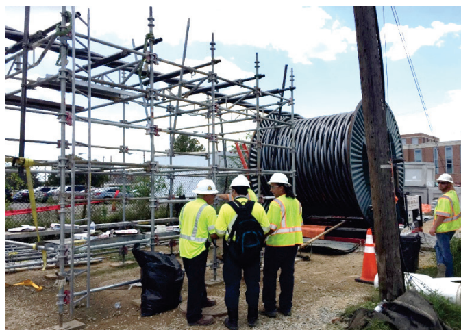
Figure 5: Preparing for cable pull.
