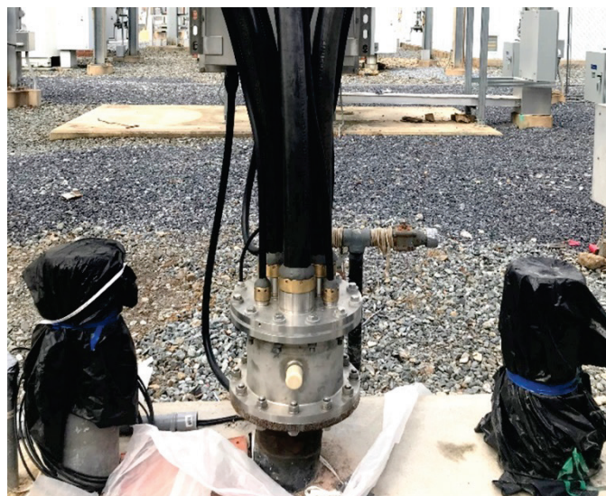
Figure 3: Trifurcation assembly for extruded cables with sealing system
